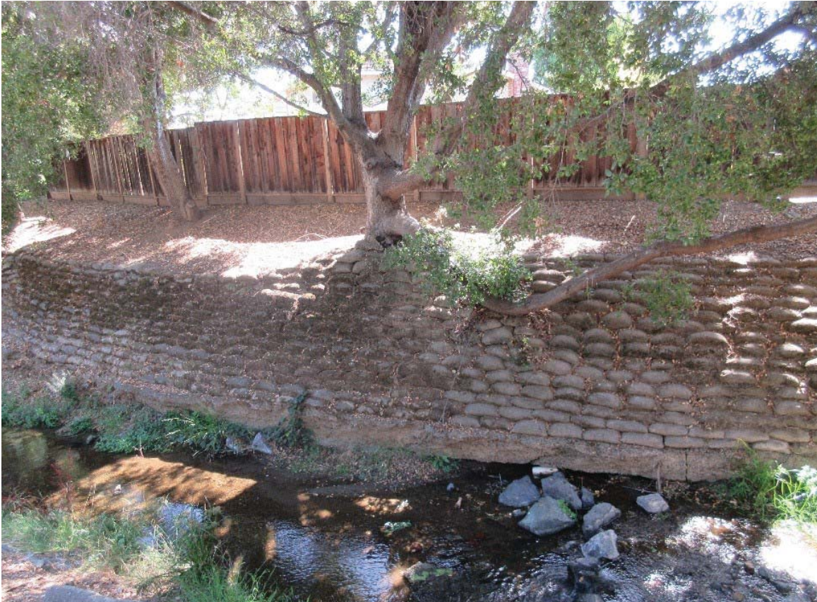
Photo 3 Sacked concrete stabilization of south side of the creek, south of Rodrigues Avenue.
