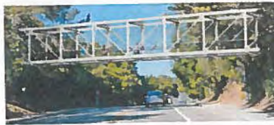
Option 2: Steel Pratt Truss Bridge
