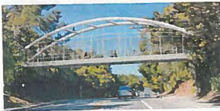
Option 4: Steel Tied Arch Bridge
