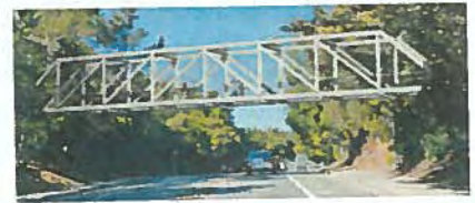
Option 3: Steel Howe Truss Bridge
