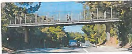
Option 1: Steel Girder Bridge
