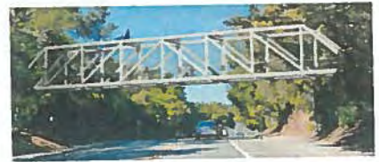
Option 3: Steel Howe Truss Bridge
