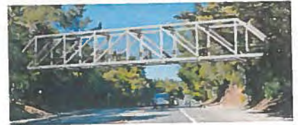
Option 3: Steel Howe Truss Bridge
