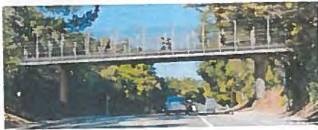
Option 1: Steel Girder Bridge
