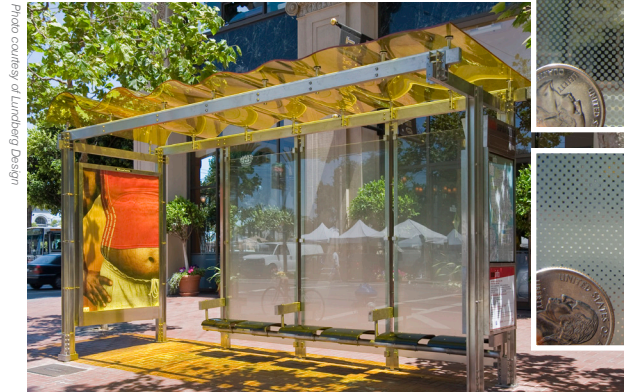
ABOVE: The City's new bus shelters designed by Lundberg Design use a subtle frit pattern to indicate the barrier. This design, called "SF Fog," is effective in alerting both people and birds to the glass. INSETS show how the frit pattern is more dense at the bottom and dissipates like the City's fog at the top.
