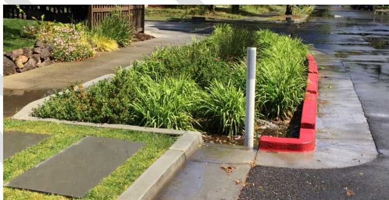
Figure 2-1 Stormwater curb extension, Southgate Neighborhood, Palo Alto (Source: EOA)
