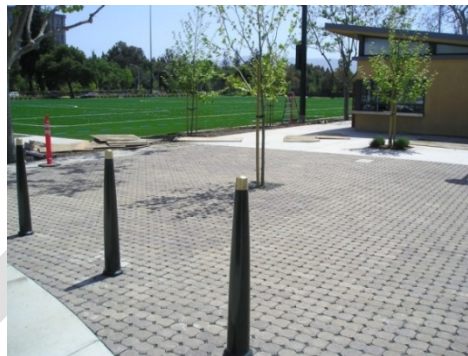
Figure 2-4 Permeable interlocking concrete pavers, Mayfield Playing Fields, Palo Alto (Source: EOA)
