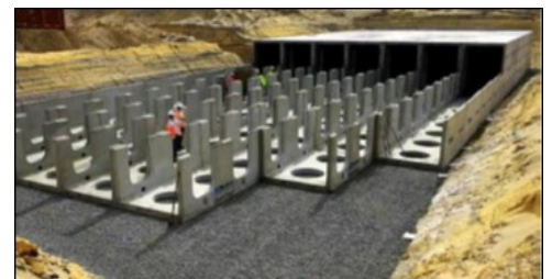
Figure 2-9 Subsurface vault, under construction (Source: Conteches.com)
