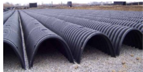
Figure 2-6 Subsurface infiltration system (Source: Conteches.com)
