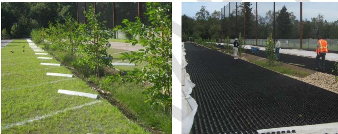
Figure 2-10 Completed green parking bays (above left) and parking bays under construction, showing the recycled plastic geocells that support vehicle weight (above right). (Source: City of Cupertino)
