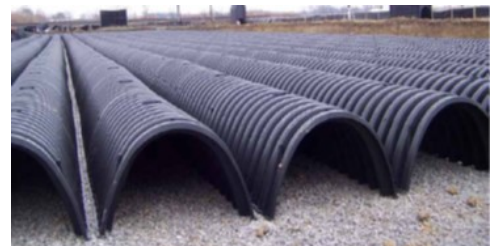
Figure 2-6 Subsurface infiltration system (Source: Conteches.com)
