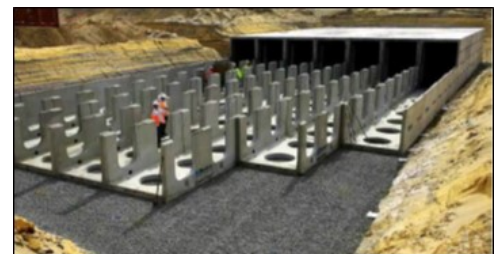
Figure 2-9 Subsurface vault, under construction (Source: Conteches.com)
