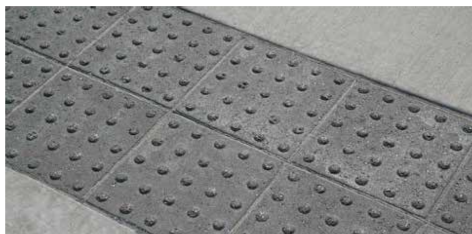
4 TRUNCATED DOMES (ON SITE) N.T.S. PHOTO
