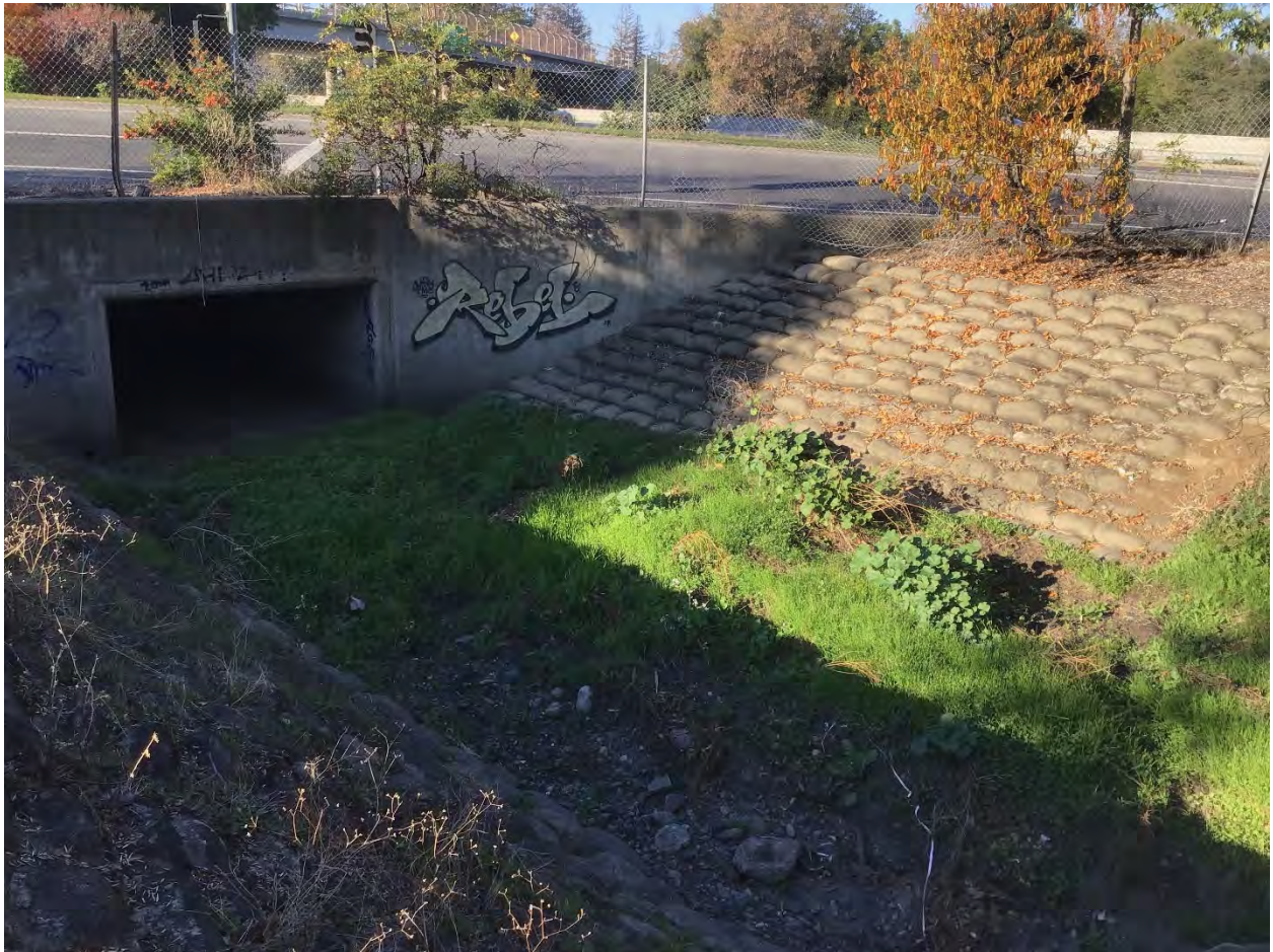
Photo 5. The Junipero Serra Channel, between Wolfe Road and Calabazas Creek, is a vegetated engineered earthen channel.
