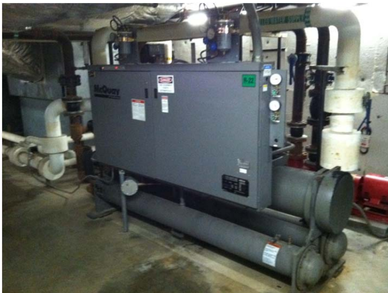
Figure 5B (Water-cooled 70 Ton Chiller)
