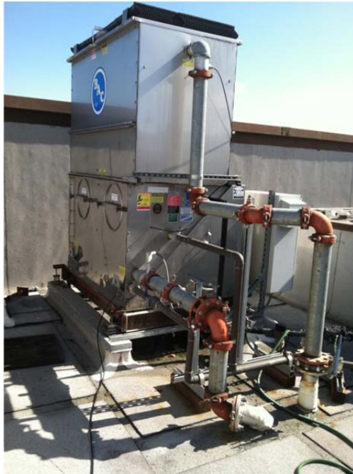
Figure 5A (Closed-Circuit 70 Ton Cooling Tower)
