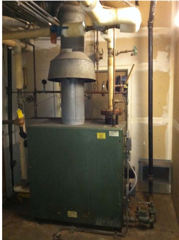
Figure 5C (Gas Fired Boiler)
