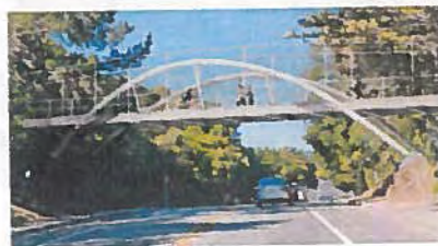
Option 5: Steel Inclined Arch Bridge
