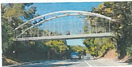
Option 4: Steel Tied Arch Bridge
