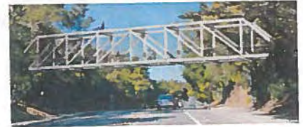
Option 3: Steel Howe Truss Bridge
