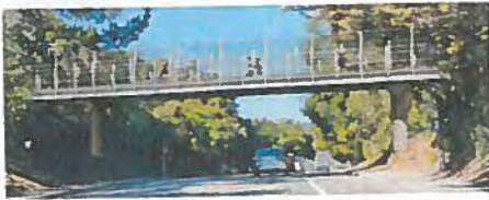
Option 1: Steel Girder Bridge
