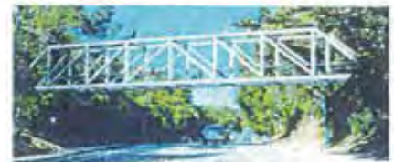
Option 3: Steel Howe Truss Bridge
