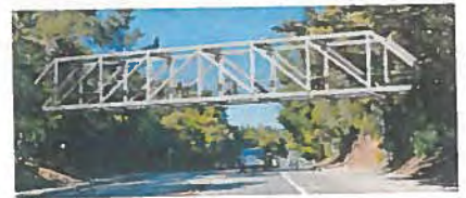
Option 3: Steel Howe Truss Bridge
