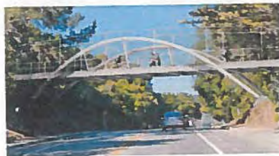
Option 5: Steel Inclined Arch Bridge
