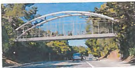
Option 4: Steel Tied Arch Bridge
