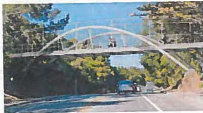
Option 5: Steel Inclined Arch Bridge
