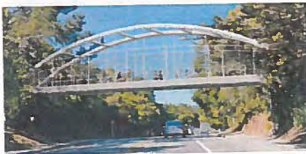
Option 4: Steel Tied Arch Bridge
