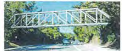
Option 3: Steel Howe Truss Bridge
