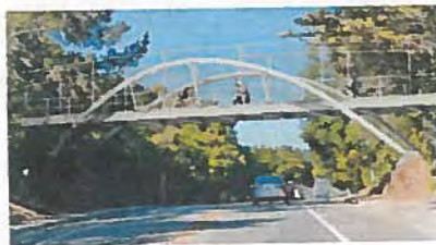
Option 5: Steel Inclined Arch Bridge
