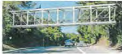
Option 2: Steel Pratt Truss Bridge
