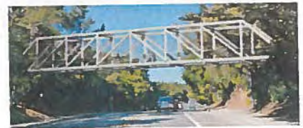
Option 3: Steel Howe Truss Bridge
