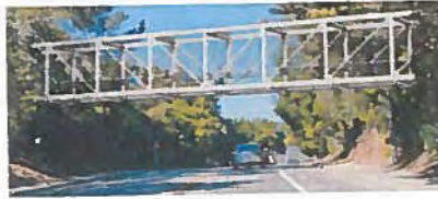
Option 2: Steel Pratt Truss Bridge
