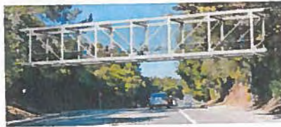
Option 2: Steel Pratt Truss Bridge
