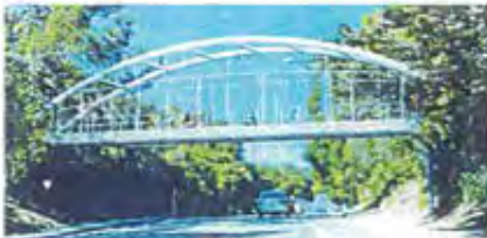
Option 4: Steel Tied Arch Bridge
