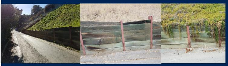
Replace failing retaining wall lagging with City forces
