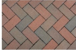
Material #4: Walkway Pavements Bricks
