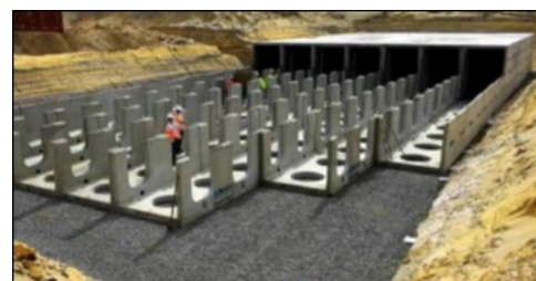
Figure 2-9 Subsurface vault, under construction (Source: Conteches.com)
