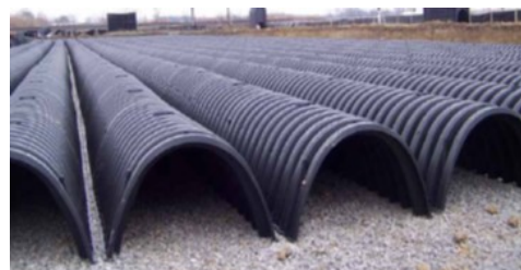
Figure 2-6 Subsurface infiltration system (Source: Conteches.com)
