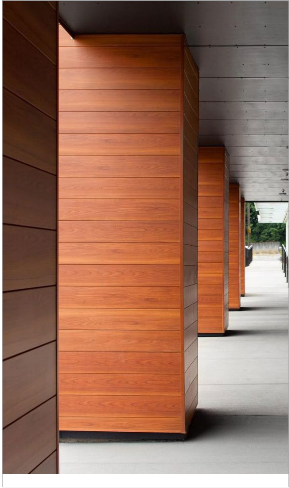
Longboard Siding - Western Cedar Installation example
