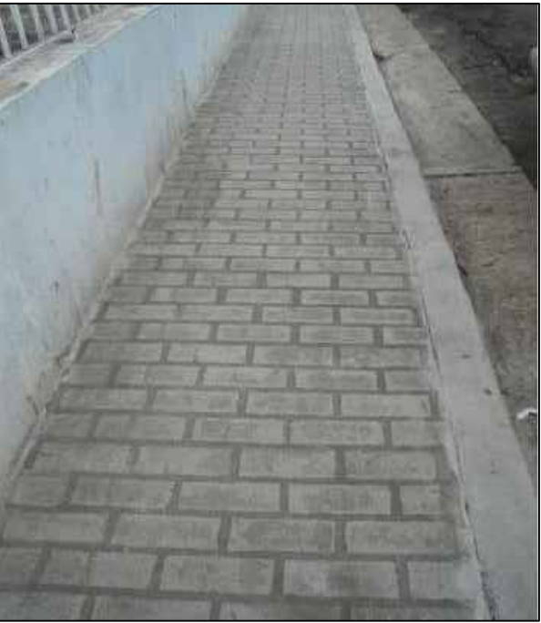
DECORATIVE CONCRETE STAMPED PATTERN: RUNNING BOND BRICK COLOR: 'DAVIS' INTEGRAL COLOR #860 'COBBLESTONE'
