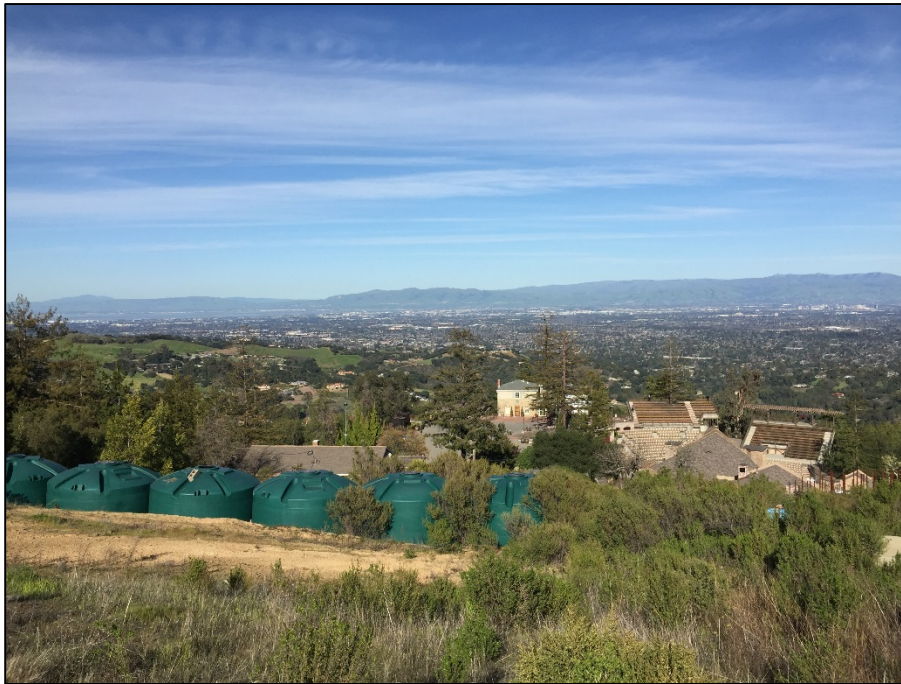
Figure 3.6. Water storage tanks at the Mountain Winery in Saratoga Hills.
