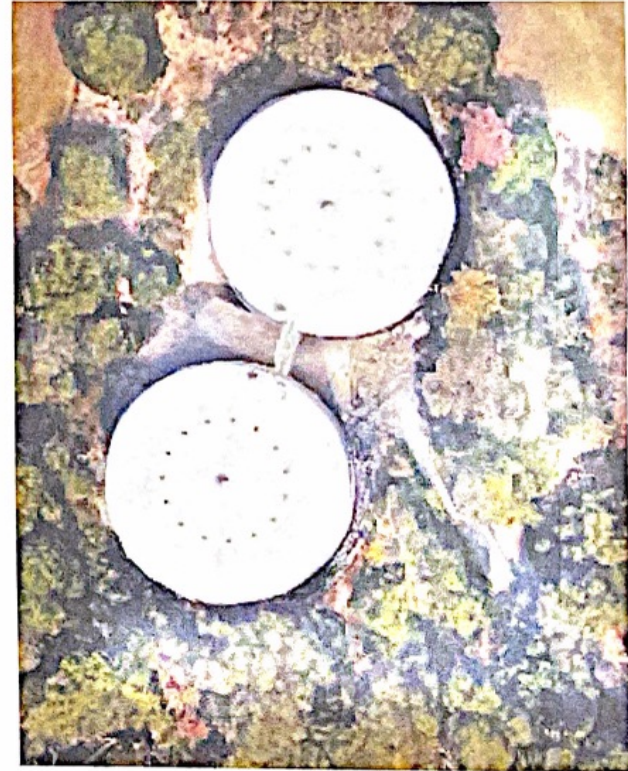
Water Utility Water Tanks
