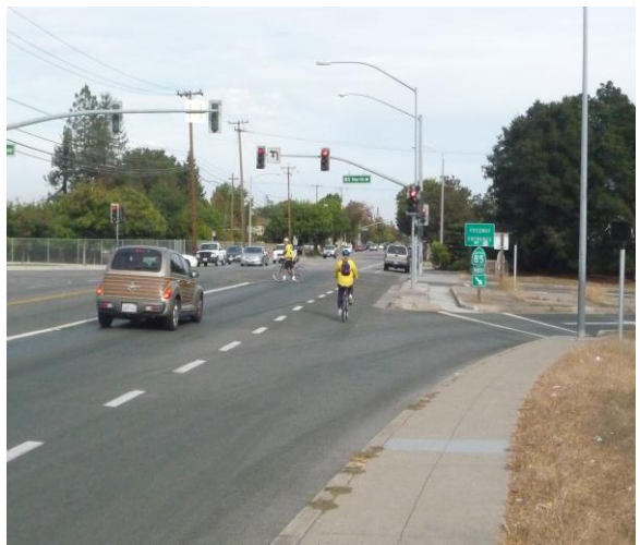
Figure 7 – Eastbound Homestead Road Approaching Bernardo Avenue/NB SR 85
