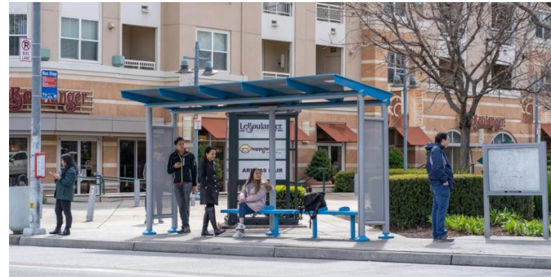
Figure 9: Rapid 523 Stop Enhancements at De Anza Boulevard
