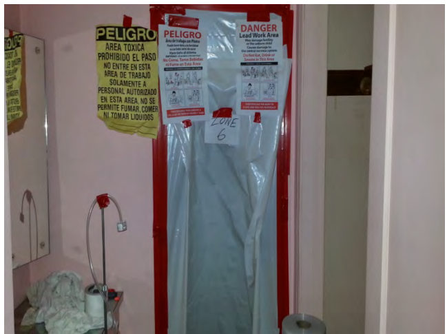
Zone 6 preparation at northeast restroom near garage
