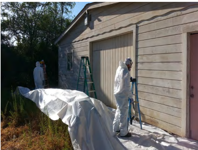
Zone 1 exterior paint scraping at the shop and outbuildings
