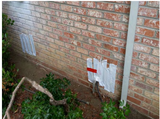
Zone 3 preparation of basement/crawlspace vents to isolate containment
