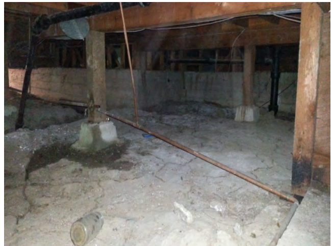
Zone 3 post removal view of crawlspace showing view of hard pan dirt floor after HEPA vacuuming
