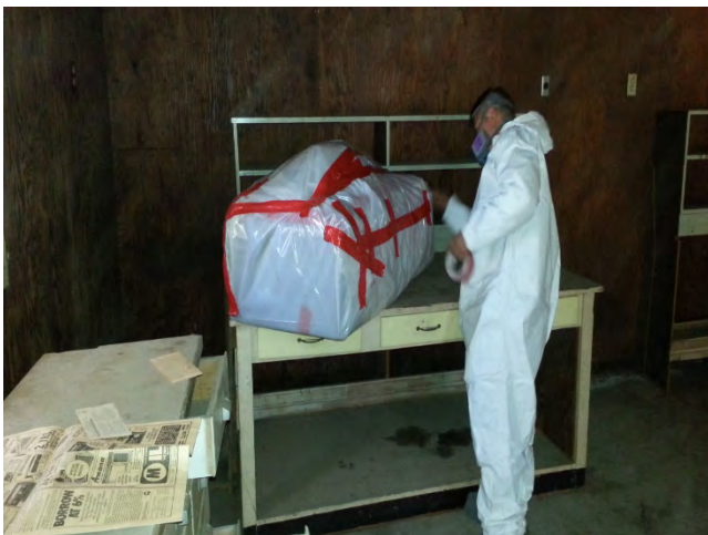
Zone 4 final wrapping of heater
