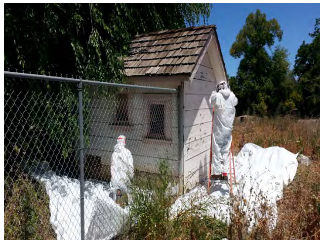
Zone 1 exterior paint scraping at the central shed
