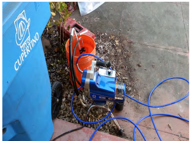
Zone 2 airless sprayer used to wet flooring materials and suppress airborne dust during removal
