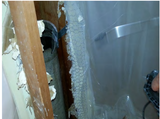
Zone 5 empty wall cavity in west wall of dining room after transite pipe removal
