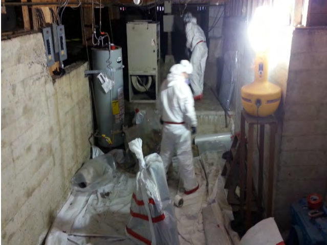
Zone 3 air scrubbing air filtration machine located in staging area of basement
