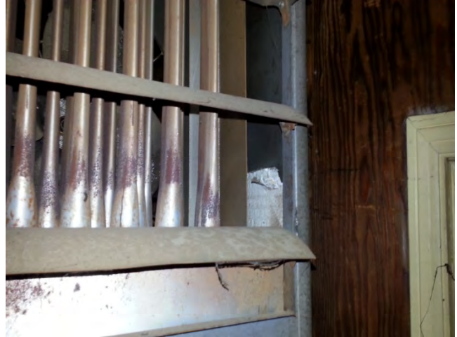
Zone 4 view of heater after being wrapped in 2 layers of 6 millimeter polyethylene sheeting before removal
