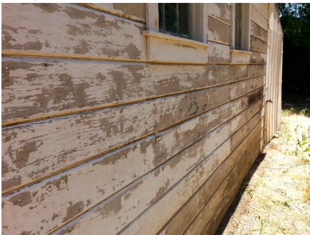
Zone 1 post removal surface of the shop following paint scraping
