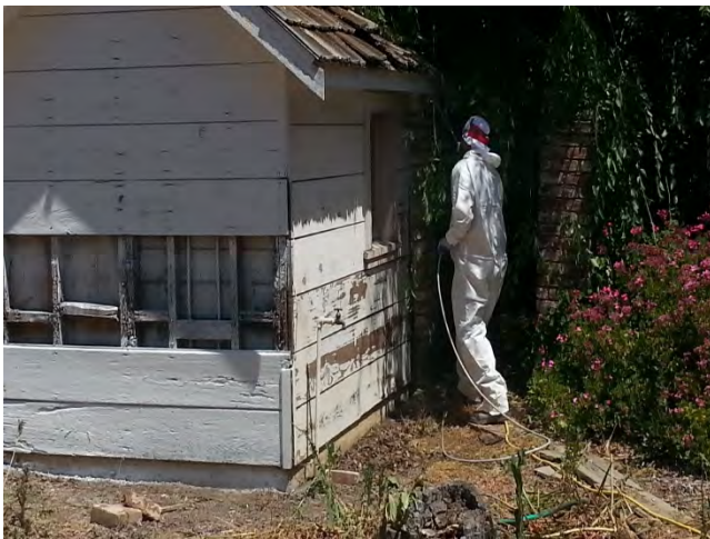
Zone 1 post removal surface of the shop following paint scraping
