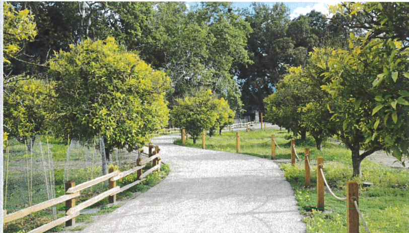
Pervious concrete application
