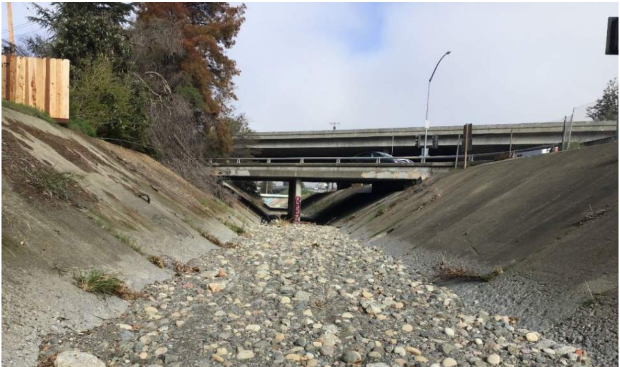
Photo 8. Engineered channel at the north end of Saratoga Creek. Moorpark Avenue Bridge in the background.
