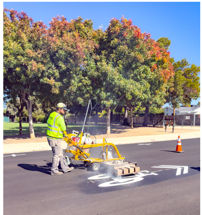
Figure 53: Sharrow installation on Pacifica Drive
