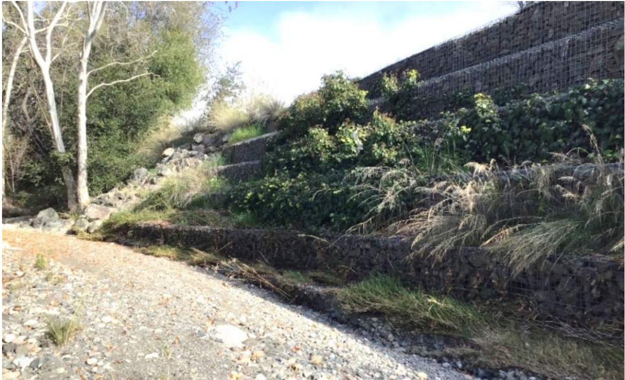
Photo 7. Gabion walls along the east bank of Saratoga Creek.
