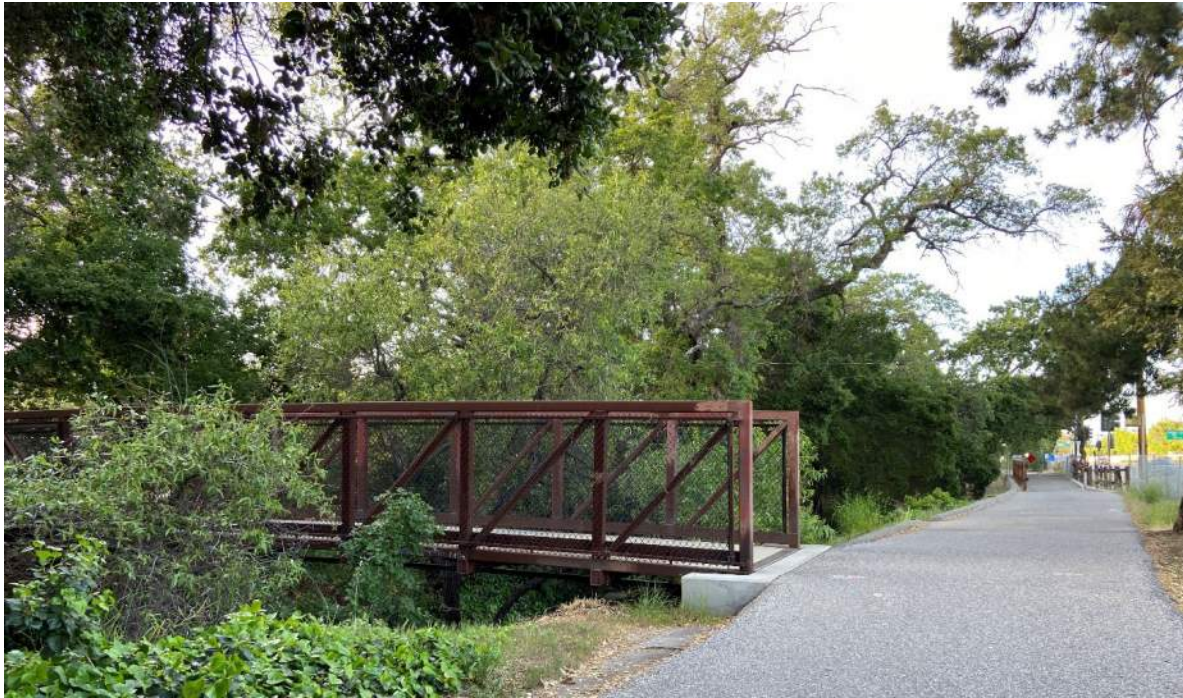
Photo 9. Pedestrian Bridge and paved trail.
