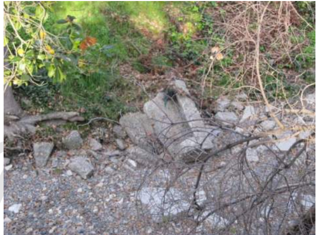
Photograph 8. Concrete debris in Saratoga Creek channel.
