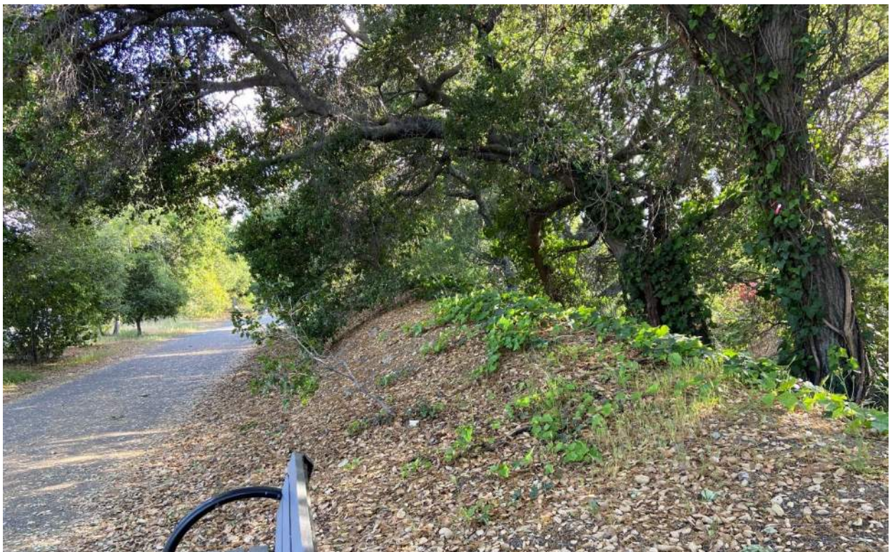
Photo 4. Berm along Saratoga Creek in the southern portion of the study area.
