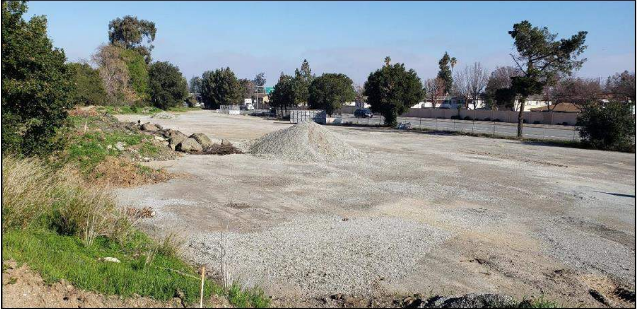
Photo 3. Viewing northeast across the site from atop the berms along Saratoga Creek.
