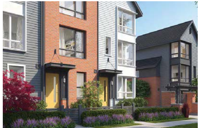
A series of dooryards with low fences defining the private edge, and engaging the sidewalk.
