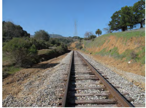
The UPRR Rail line runs between Rancho San Antonio County Park and Stevens Creek Boulevard.
