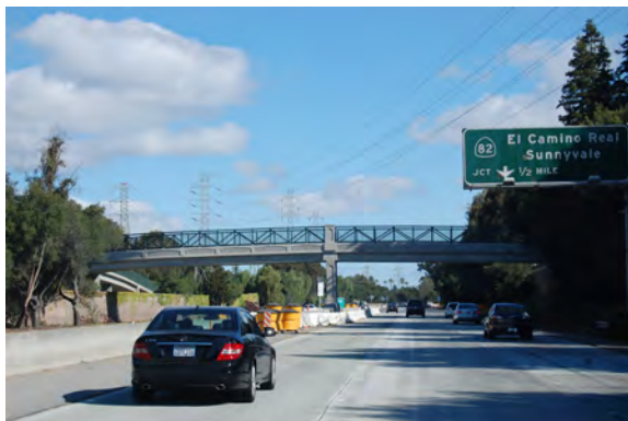
Pedestrian overcrossing at State Route 85 in Mountain View.
