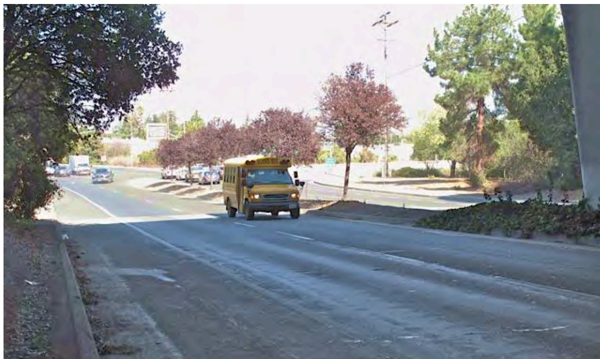
Foothill Expressway beneath Interstate 280.
