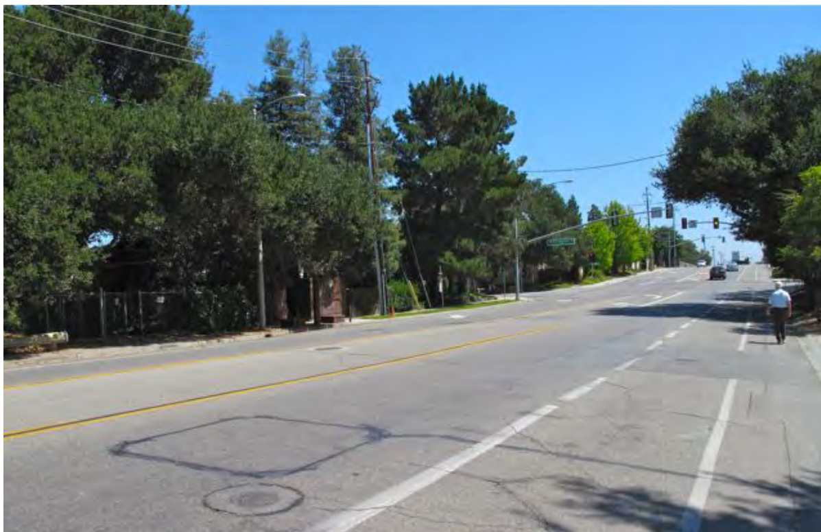
Homestead Road was one of many streets assessed for closing the gap in the Stevens Creek Trail.
