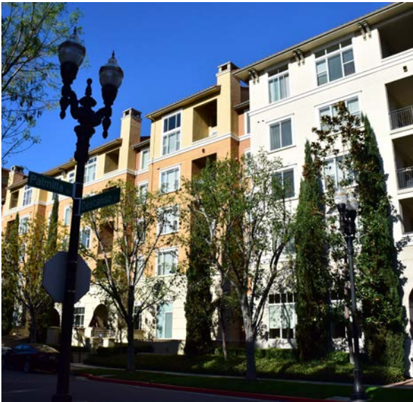
North Park Apartments, San Jose
