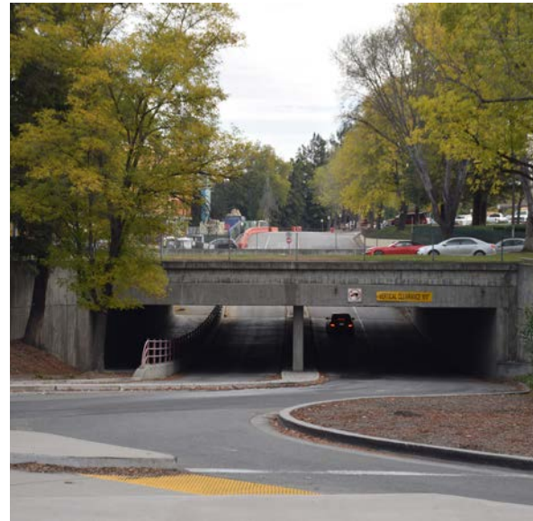
Perimeter Road east-west underpass beneath North Wolfe Road
