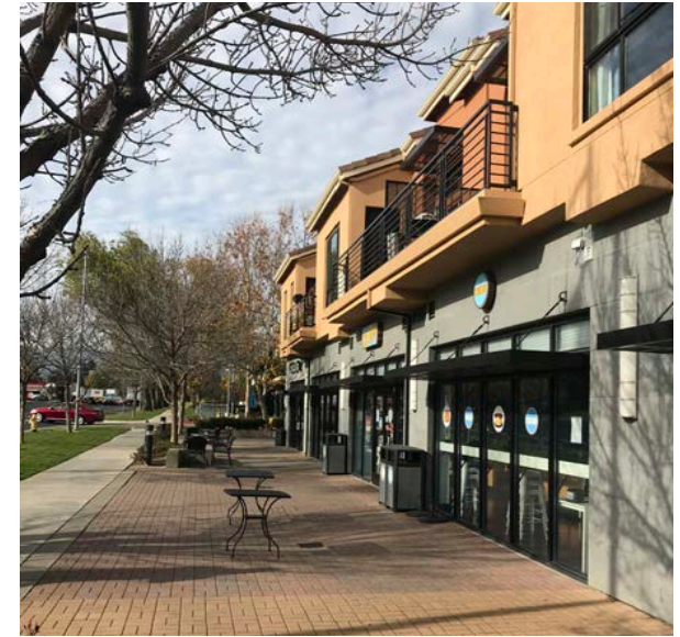
Mixed-Use with Shopfronts at Metropolitan Condos
