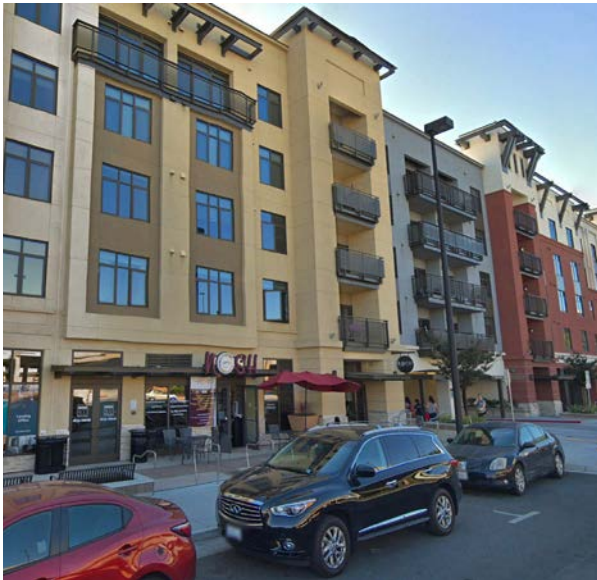
Mixed-Use Shopfronts, Nineteen800
