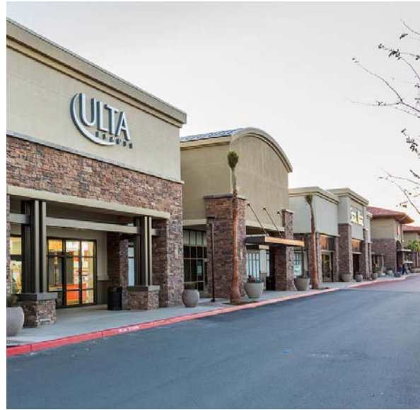
Homestead Square, Cupertino
