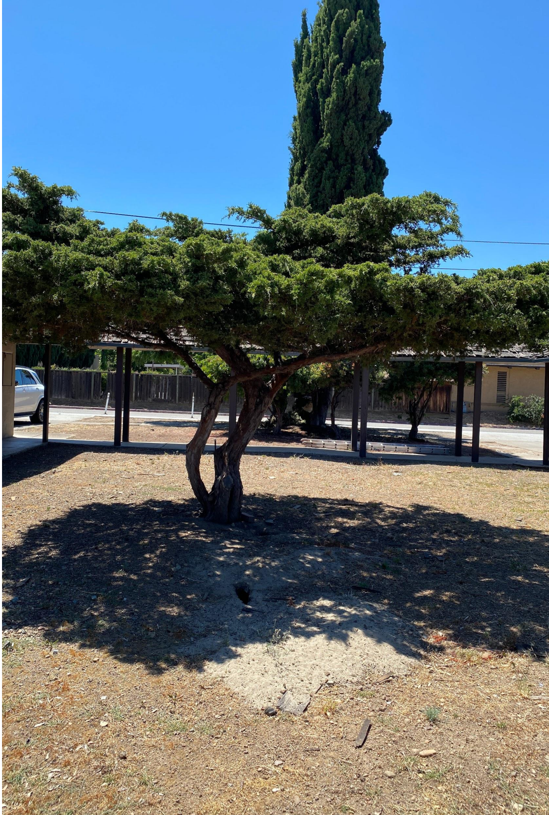
Photo 4. Tree #7 is in good condition but is in the footprint of the planned construction and will require removal
