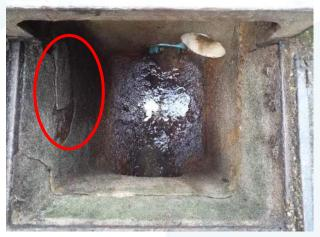
Photo 31. Concrete spalling and moderate cracking of SWST4473 (VANDA Level 3).
