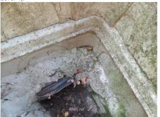
Photo 29. Moderate surface damage in SWST434 (VANDA Level 3).
