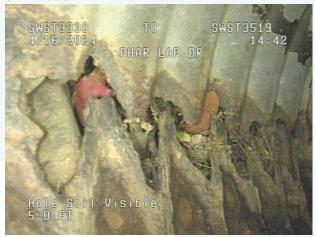
Photo 4. Grade 5 structural defect on CMP (hole); SWPP1698.
