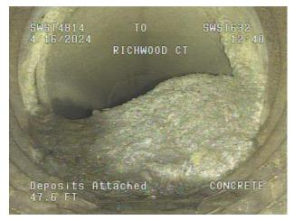
Photo 11. O&M Grade 4 defect due to concrete deposits; SWPP1546
