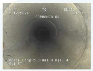
Photo 2. Crack longitudinal hinge on RCP, (Grade 4); SWPP4745.
