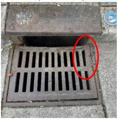
Photo 27. Broken catch basin cover; SWST2015 (VANDA Level 4).
