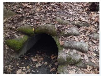
Photo 24. Minor surface damage to outfall structure SWST3549 (VANDA Level 2).
