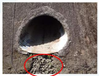
Photo 19. Spalling of outrall structure SWST26153 (VANDA Level 3).
