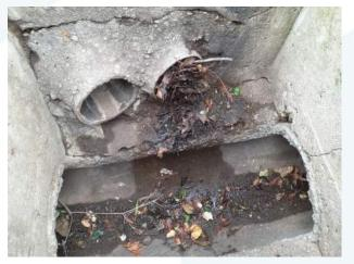
Photo 25. Frequent cracking along catch basin SWST24885 (VANDA Level 4).
