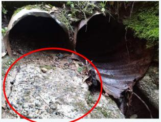
Photo 20. Moderate surface damage on outfall structure SWST25297 (VANDA Level 3).
