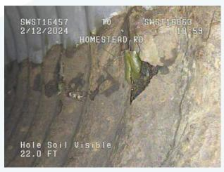
Photo 8. Hole in CMP pipeline due to corrosion (Grade 5); SWPP4896.
