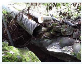
Photo 14. Large cracking of outfall structure; undermining (VANDA Level 5); SWST25337.
