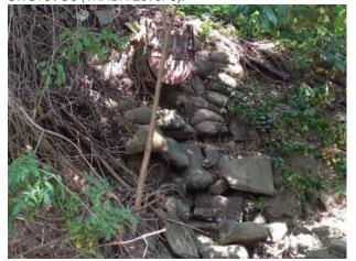
Photo 17. Severe damage to outfall headwall SWST4805 (VANDA Level 4).
