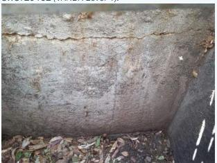
Photo 28. Moderate crack in structure SWST3066 (VANDA Level 3).
