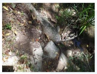
Photo 13. Collapsed outfall structure SWST3548 (VANDA Level 5).
