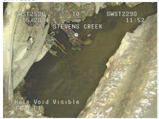
Photo 6. Grade 5 structural defecton CMP (large hole/void); SWPP3360.
