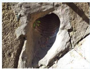
Photo 22. Moderate surface damage and cracking of outfall structure SWST3528 (VANDA Level 3).
