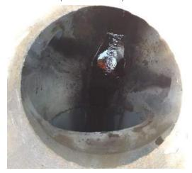
Photo 35. Minor surface damage of SWST1179 (VANDA Level 2).
