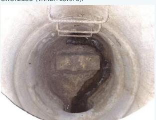
Photo 34. Minor surface damage SWST2412 (VANDA Level 2).
