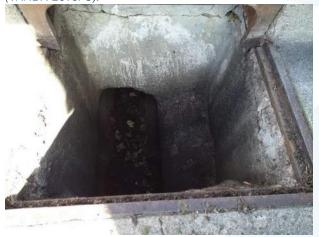
Photo 30. Moderate cracking of SWST1411 (VANDA Level 3).
