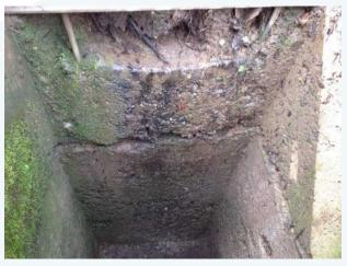
Photo 26. Moderate surface damage and voids in SWST10461 (VANDA Level 4).
