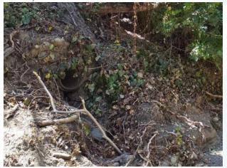
Photo 18. Severe damage to outfall headwall SWST4807 (VANDA Level 4).
