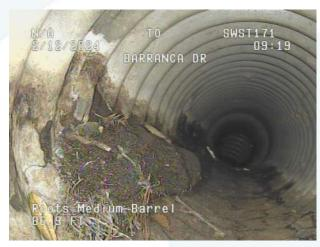
Photo 7. Hole with soil visible on CMP (VANDA Level 5); SWPP4745.
