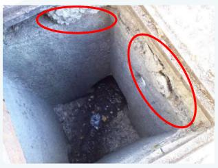
Photo 32. Deterioration of concrete under cover frame in SWST2156 (VANDA Level 3).
