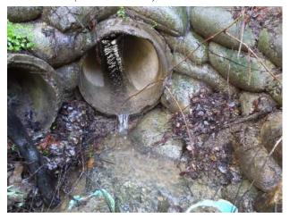
Photo 23. Minor surface damage to outfall structure SWST433 (VANDA Level 2).
