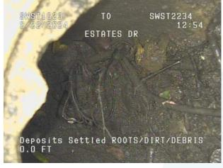
Photo 12. Grade 5 defect due to roots, dirt, and debris; SWPP3283.
