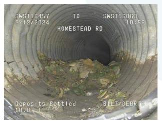
Photo 3. Grade 4 structural defect on CMP; Grade 3 O&M defect (debris); SWPP4896.
