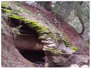
Photo 15. Failure of the headwall and undermining at SWST3786 (VANDA Level 5).
