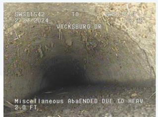
Photo 10. 0&M Grade 5 defect due to debris; SWPP3661.
