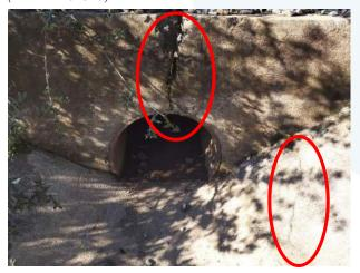
Photo 21. Moderate cracking of outfall structure SWST26153 (VANDA Level 3).
