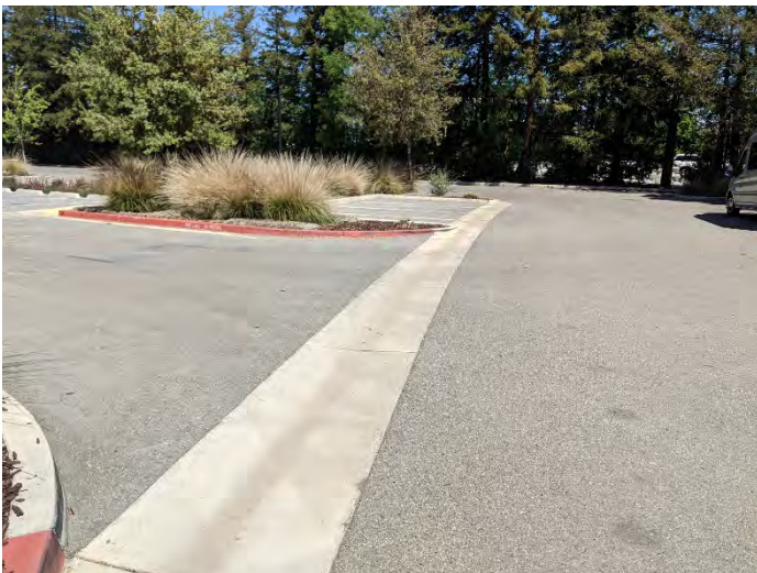
Photo 15: View of typical concrete surface water drainage in parking lot.
