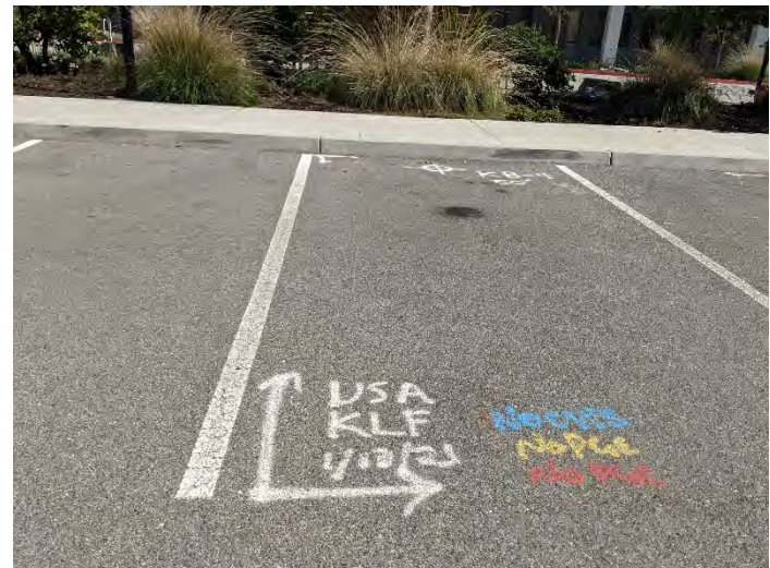
Photo 18: Evidence of previous subsurface investigations (possible geotechnical drilling) on the Subject Property.
