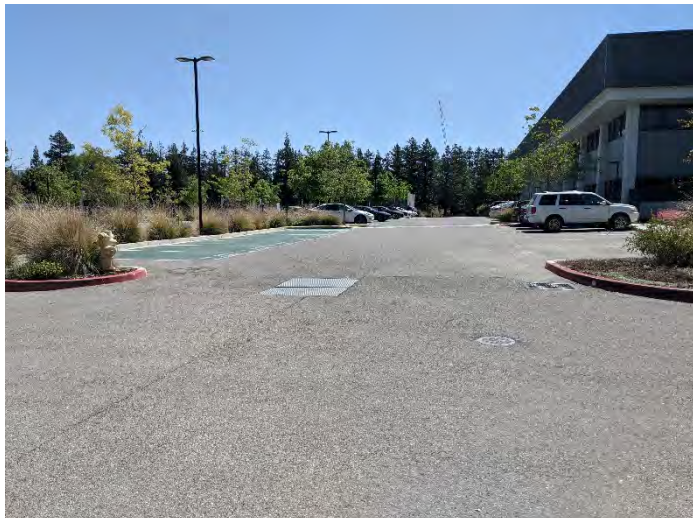
Photo 3: View of driveway adjacent to north side of Subject Property building, looking southeast.
