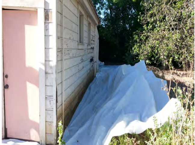
Zone 1 preparation measures for lead paint removal and stabilization at the shop
