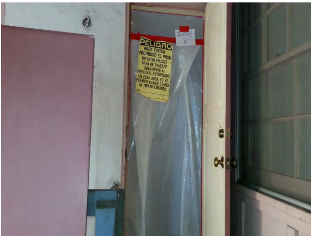
Zone 6 preparation showing HEPA exhaust tubing at master bathroom
