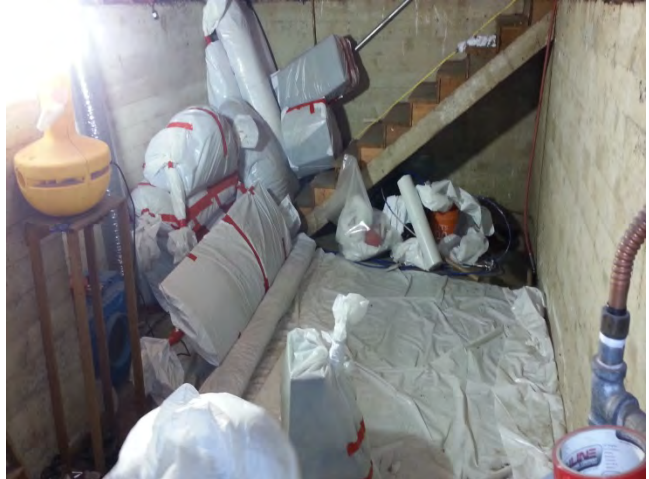
Zone 3 workers wrapping HVAC ductwork in polyethylene sheeting
