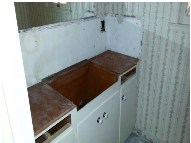
Zone 6 northwest guestroom counter following removal of ceramic tile counter
