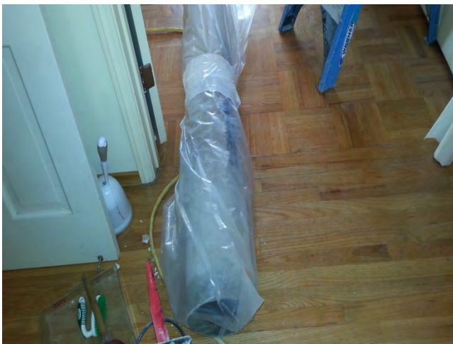
Zone 5 five foot section of transite pipe wrapped in 2 layers of polyethylene sheeting after removal
