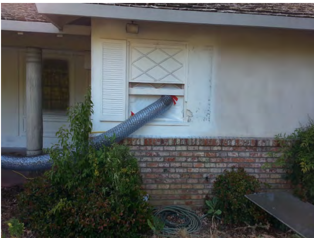
Zone 6 preparation showing HEPA exhaust tubing at master bathroom
