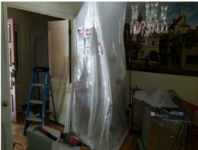
Zone 5 five foot section of transite pipe wrapped in 2 layers of polyethylene sheeting after removal
