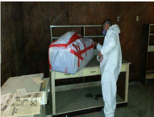
Zone 4 final wrapping of heater
