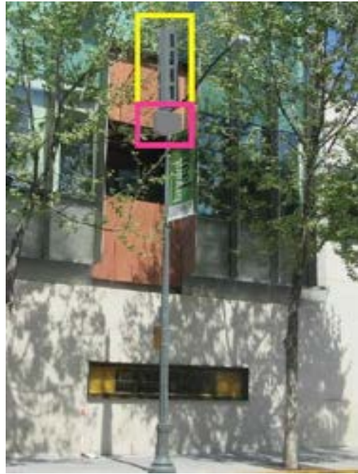
Figure 8: Stand-alone small cell poles (as shown in this example) are not preferred but may be permitted if enclosure of all equipment within the pole or in an underground vault is technically infeasible.
