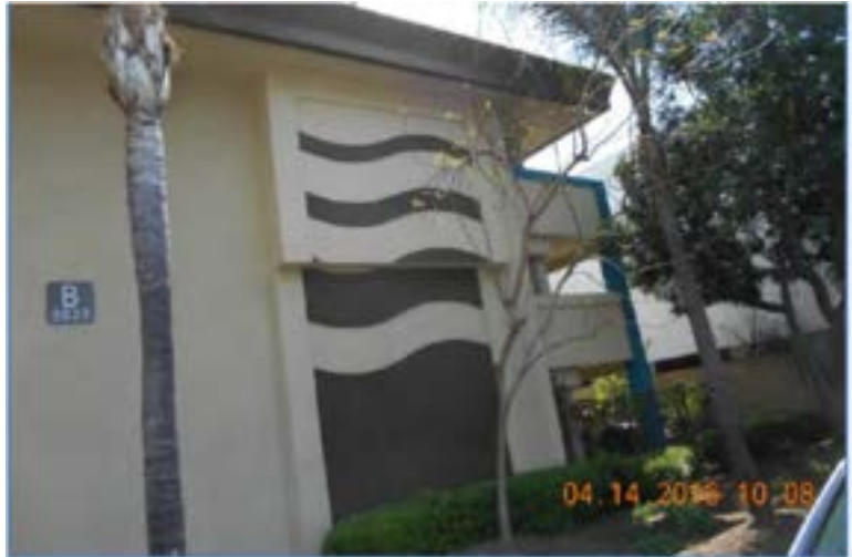
Figure 5: Although façade-mounted boxes are not preferred, this example from San Diego achieves integration with the structure.
