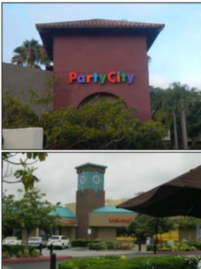
Figure 4: A cupola (above) and a clock tower (below) conceal antennas.
