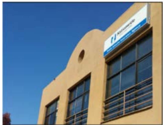
Figure 3: Antennas are concealed behind the circular element.
