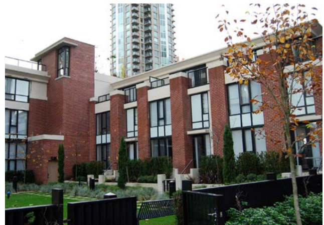
This residential forecourt provides an entry yard and breaks down the overall massing along the street.
