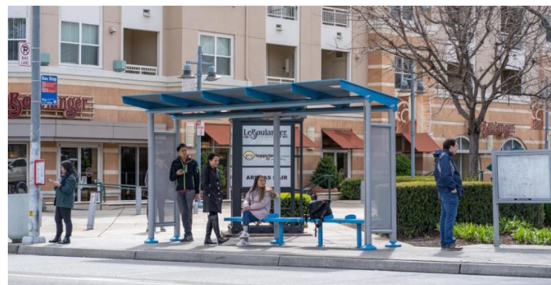
Figure 9: Rapid 523 Stop Enhancements at De Anza Boulevard
