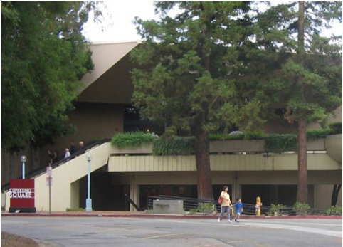
The City Council may grant height increases above the maximum base height standard in certain areas if a project includes community benefits
