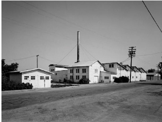
Woelffel Cannery 10120 Imperial Avenue – Demolished
