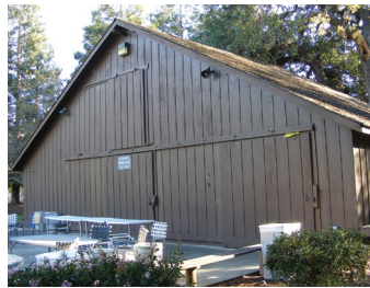
Glendenning Barn 10955 N Tantau Avenue – Hewlett Packard
