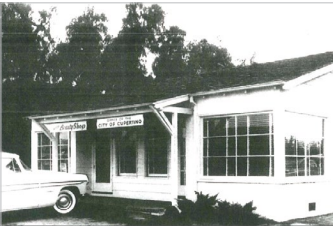
Interim City Hall 10321 South De Anza Boulevard
