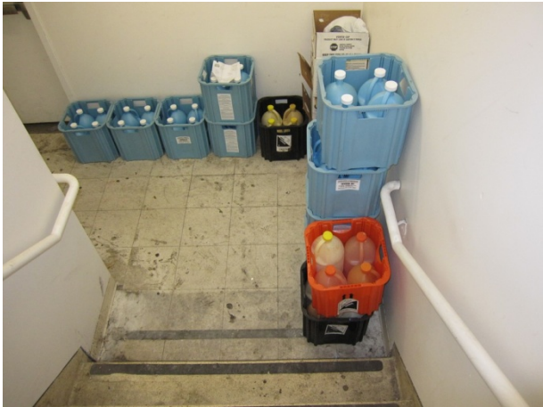
Photograph 13. Pool chemicals stored in stairwell at Bay Club.
