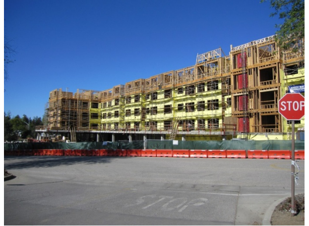
Photograph 4. Hotel under construction (APN 316-20-092).
