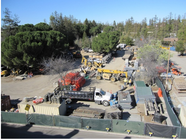
Photograph 3. Construction storage activities (APN 316-20-088).
