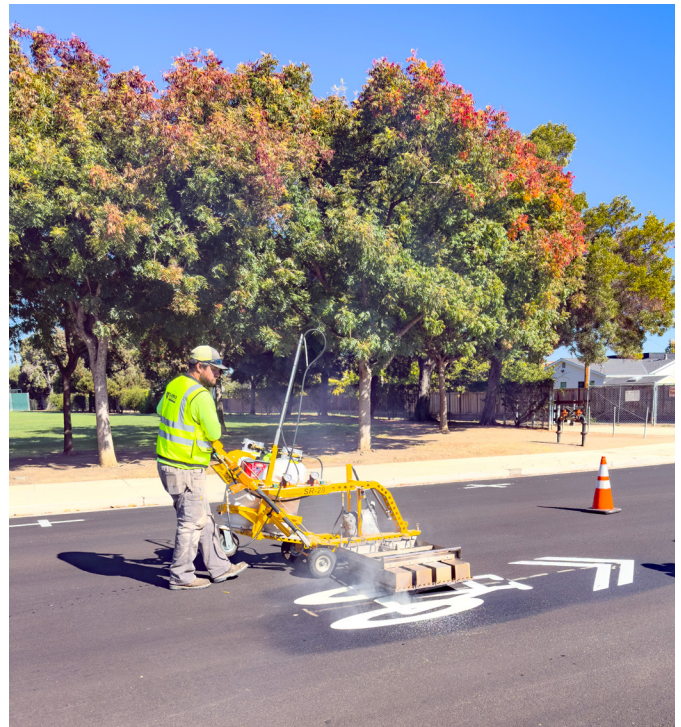
Figure 53: Sharrow installation on Pacifica Drive
