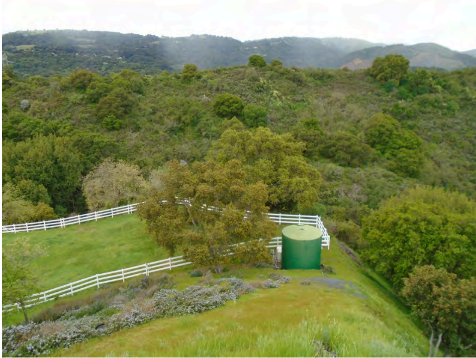
5. View of water tank on easement of subject property
