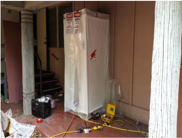
Zone 3 air filtration machine attached to HVAC opening in living room
