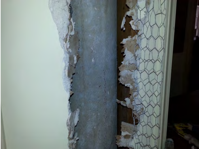
Zone 5 mini-containment constructed to isolate removal of transite pipe during work
