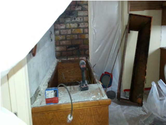
Zone 6 final condition of kitchen counter and back splash following removal of ceramic tile
