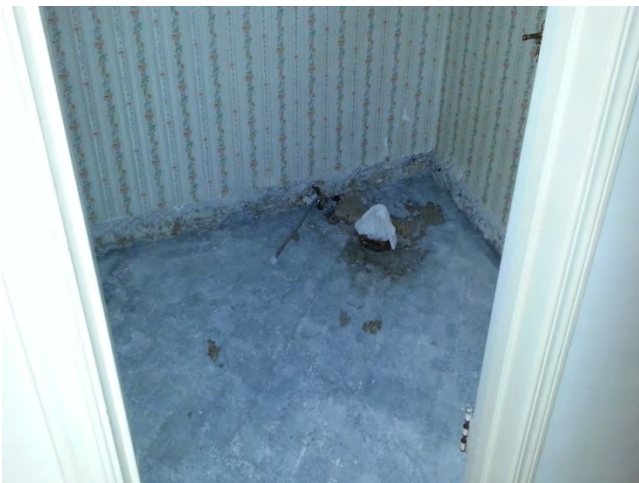
Zone 6 final condition of northeast restroom floor following removal of ceramic tile
