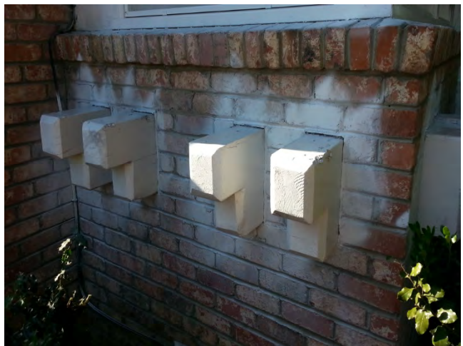
Zone 1 post removal and stabilization of the flower box shelves of the main house
