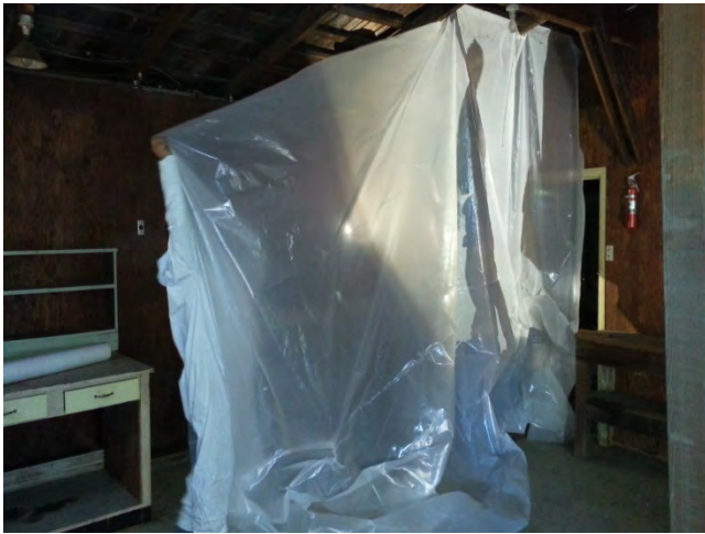
Zone 4 final wrapping of heater
