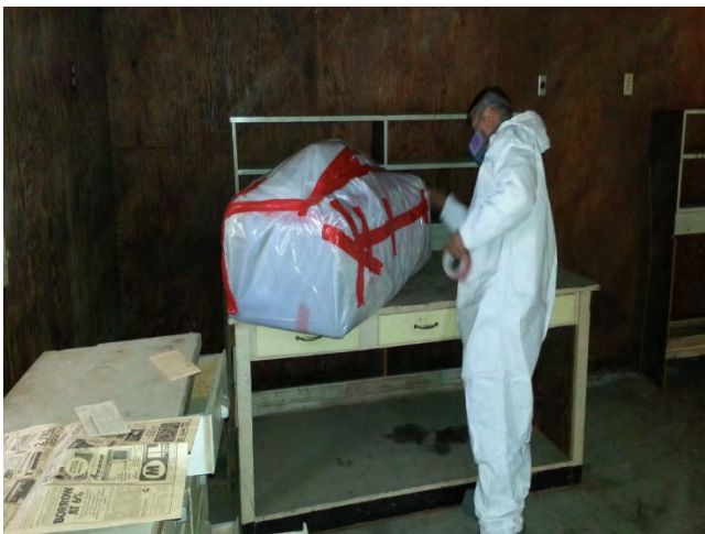
Zone 4 final wrapping of heater
