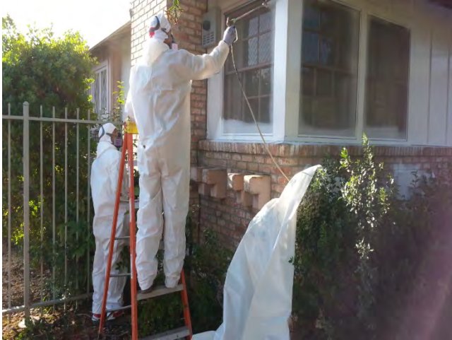
Zone 1 paint stabilization and repainting of the central shed
