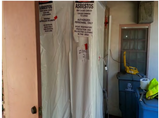
Zone 2 view of manometer recording sufficient negative air pressure inside work area
