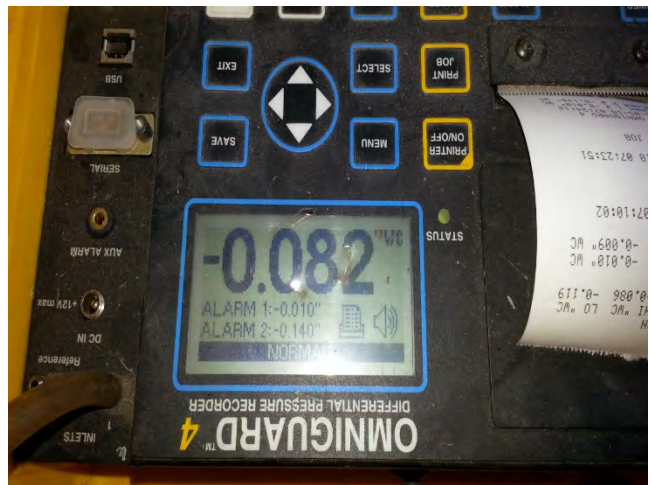
Zone 2 view of manometer recording sufficient negative air pressure inside work area
