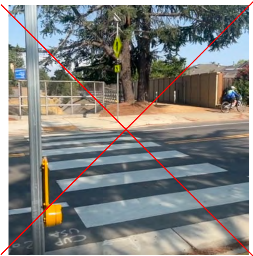
EXISTING REGNART CREEK & BLANEY CROSSWALK:
