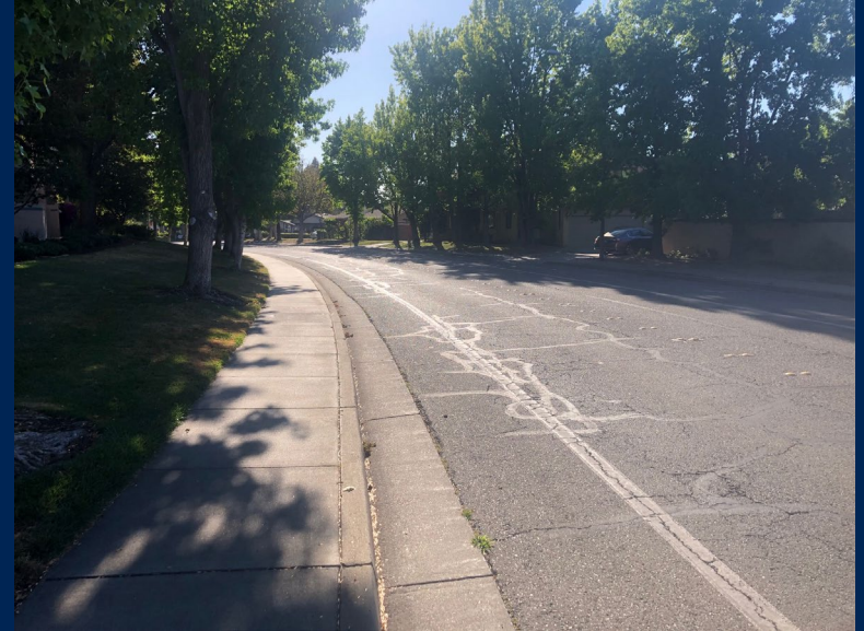
Looking to east – 240'
