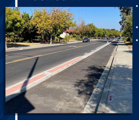
Cast-in-place concrete buffer 1.5' wide
